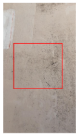
3.0 Item 15 (Picture) back patio
