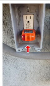
4.2 Item 1 (Picture) main panel
