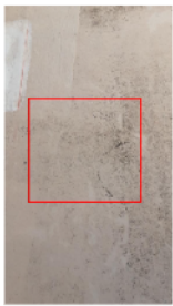
3.0 Item 15 (Picture) back patio
