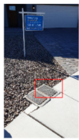
1.0 Item 1 (Picture) water meter
