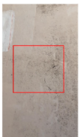
3.0 Item 15 (Picture) back patio
